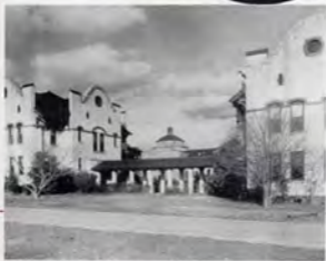
The Dome from Back Campus
