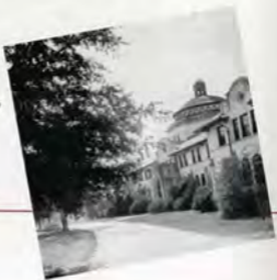
West Hall looking south
